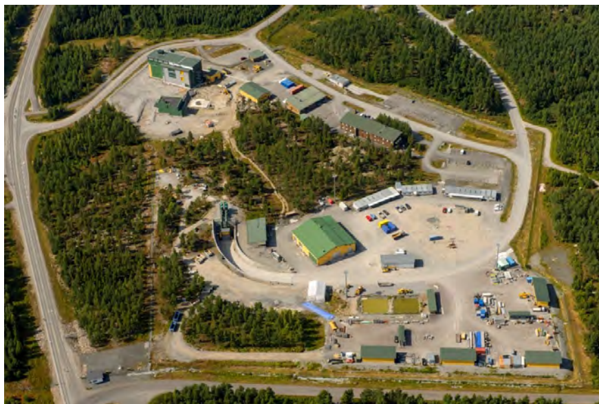
Figure 14–2 Entrance of the tunnel leading to the spent fuel final disposal research facility (ONKALO) at Olkiluoto.
