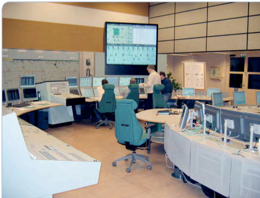
Figure 3–5 Control room of the training simulator for plant units OL1 and OL2.
