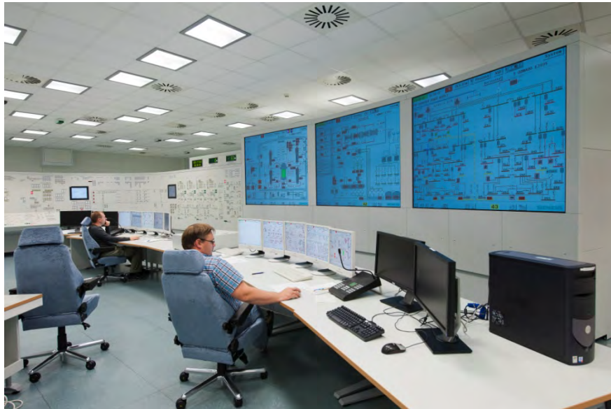
Figure 3–6 Control room of the training simulator for plant unit OL3.
